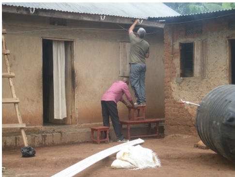
Making progress on rainwater project
