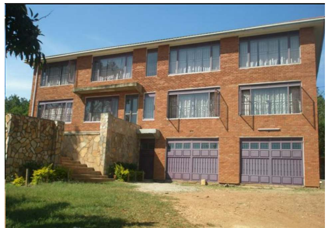
Front view of Lookout Ridge
